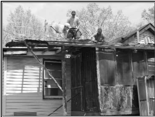
Volunteers work on exterior house improvements for HOA.
