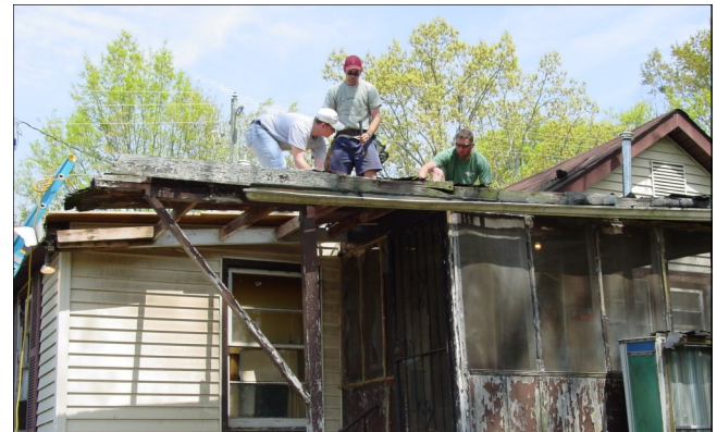
Demolition of a rear porch at 645 Dearing Street.
