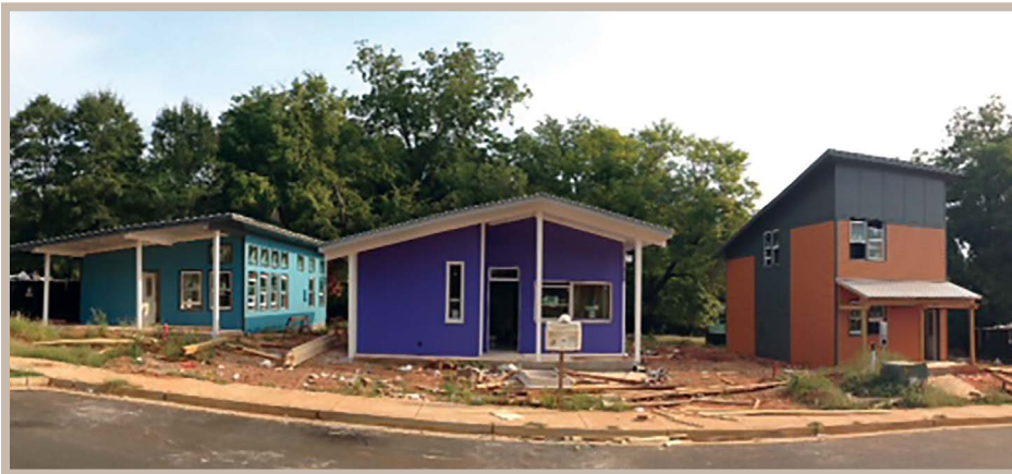
Three of the Cottages at Cannontown are under construction.
