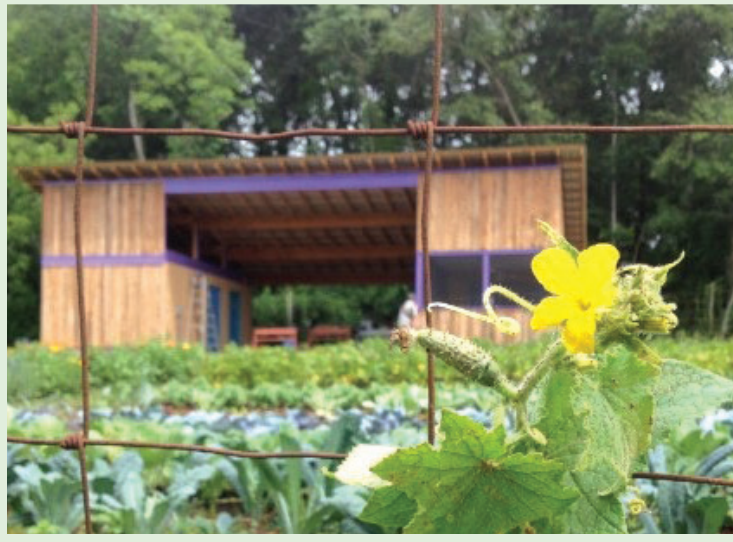
The pavilion at Williams Farm houses wash stations, walk-in cold storage, and other resources available to incubator farmers for growing, harvesting, and processing produce.
