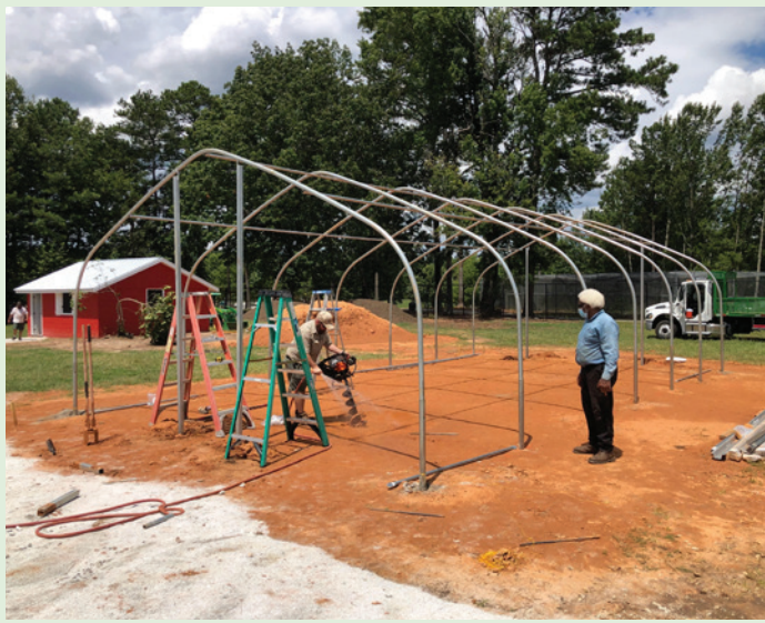
Farmer Outreach Specialist, Dr. Sherman Green, helping a grower install a hoop house that was acquired through the Environmental Quality Incentives Program. Hoop houses help farmers extend their growing seasons.
